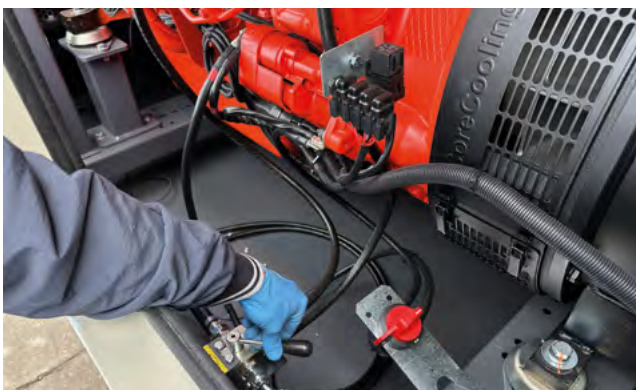
3-way valve for external tank connection
