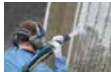
8.6 to 10 bar: Abrasive blasting
