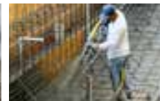
7 to 12 bar: Shotcrete applications
