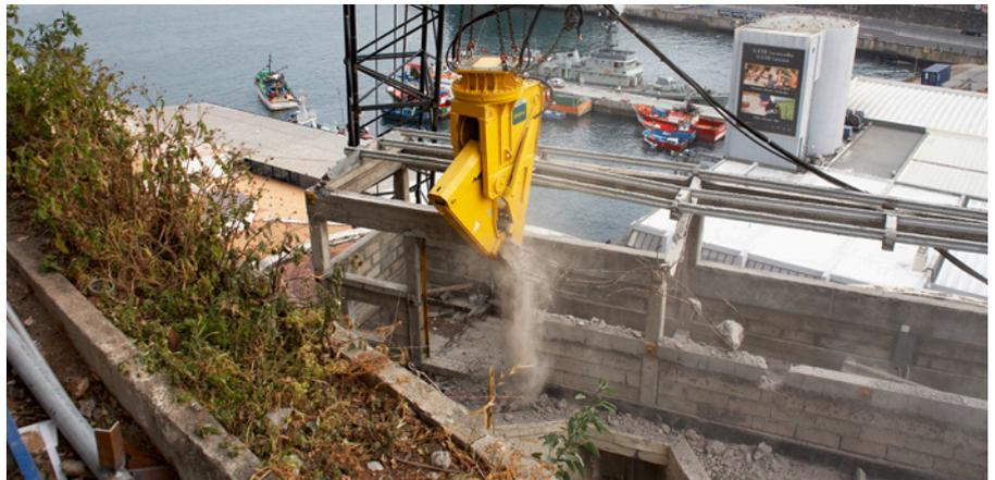
Long-term use is guaranteed by the extremely robust design of the Demolition Pulverizers. Wear parts are also easily replaced on-site.
