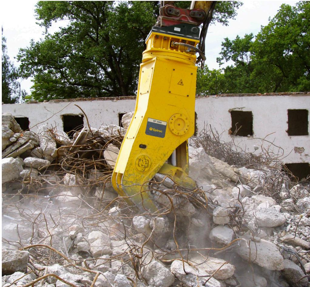
The Bulk Pulverizers' smart design also makes them ideal for primary demolition of ceilings and walls.
