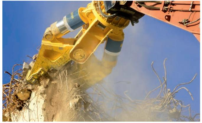
Two independently moving jaws eliminate displacement force, thus lowering stress levels.
